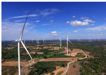
Wind Farm Power Project in Thailand
